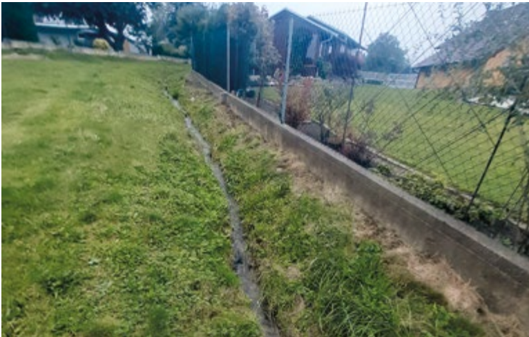
Fig. 6. Minor watercourse near the main road, standard situation (October 2024)
