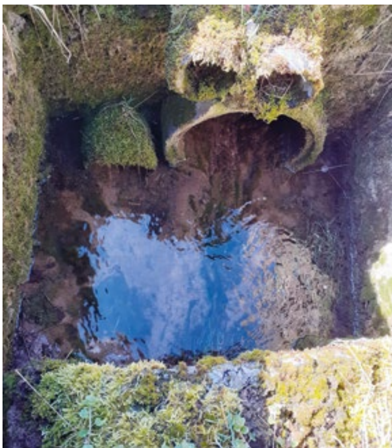
Fig. 8. Piped water flow/melioration in Šitbořský stream valley and the bottom of the future reservoir (LAPV Tuřany)
