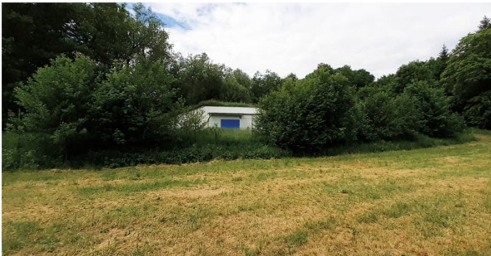
Fig. 7. Groundwater pumping facility in Šembera alluvial plain (LAPV Tuchoraz)
