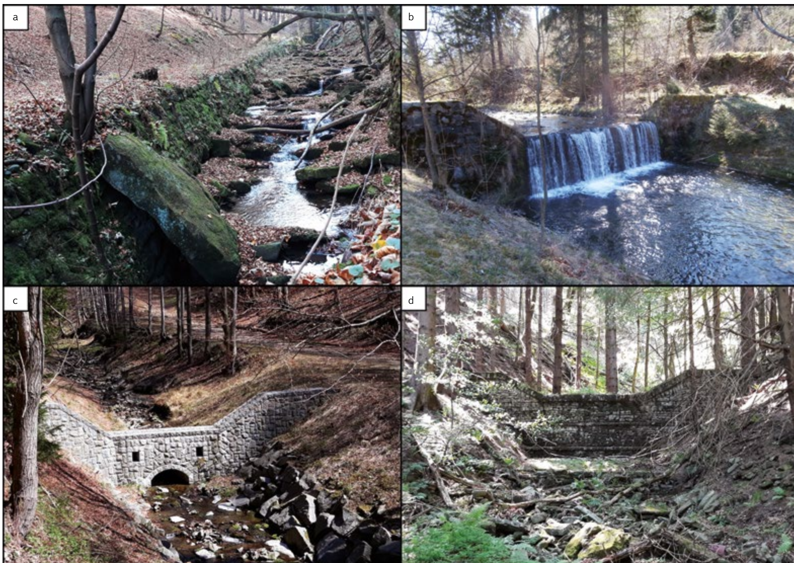
Fig. 7. Anthropogenic disconnection within the Slavíč catchment: a) old embankment on the upper part of the Slavíč stream; b) stabilization step on the lower part of the Slavíč stream; c) retention barrier built on the Ropičný stream; d) old retention barrier on the source area of the Slavíč stream
