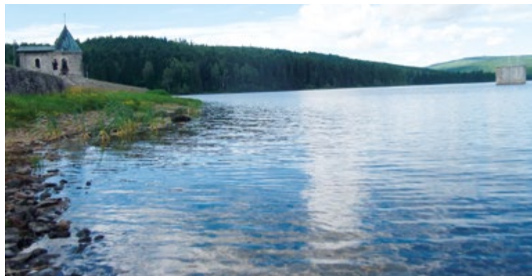
Fig. 3. Water, later drinking water reservoir Souš, built in 1915 on the Černá Desná river. The dam was reconstructed in the 1920s and 1970s, after the catastrophe of a reservoir in the parallel Bílá Desná river valley; June 2012 (Photo: D. Vondrák)
