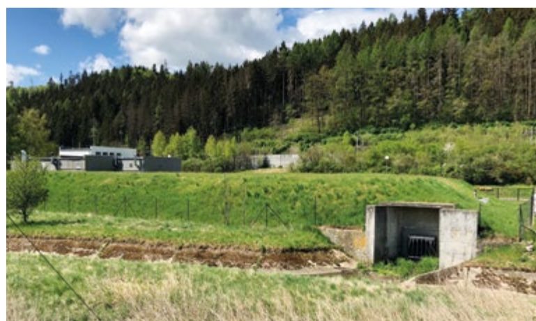
Fig. 5. An example of a ground water reservoir near the town of Březová nad Svitavou (Photo: A. Létal, May 5, 2020)
